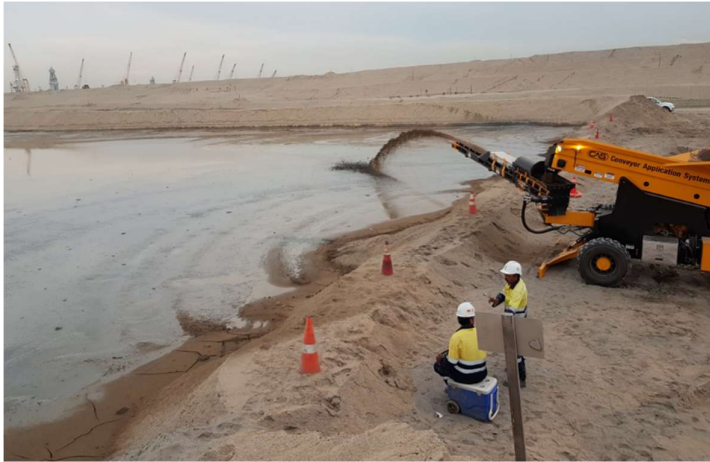
Figure 4. Sand slinger in action.
