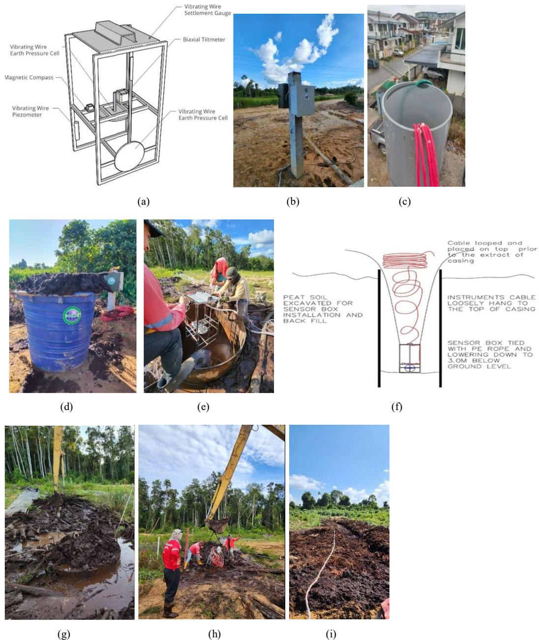
Figure 3 Sensors: (a) Sensor box, (b) Sensor reference tank and data logger placed on pile (c) Calibration cylinder, (d) Peat tank, (e) Burial of the sensors, (f) Schematic of burial process, (g) Backfilling the excavated peat, (h) Extracting the casing (i) Cable trench
