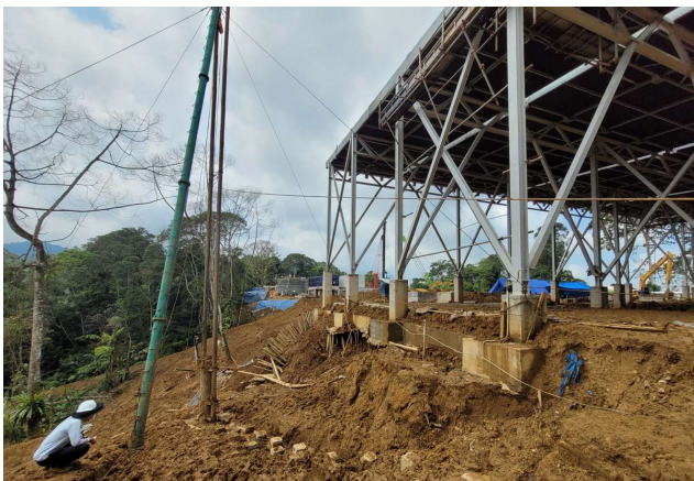
Figure 14. Pile driving work –August 2022
