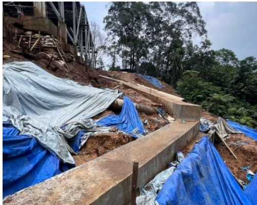
Figure 17. Geofoam installation area – November 2022
