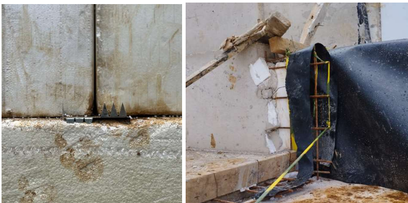
Figure 19. Gripper for interlocking and details of surface protection –December 2022
