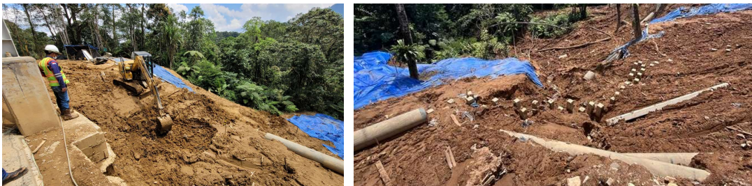
Figure 15. Pile driving work progress –September 2022
