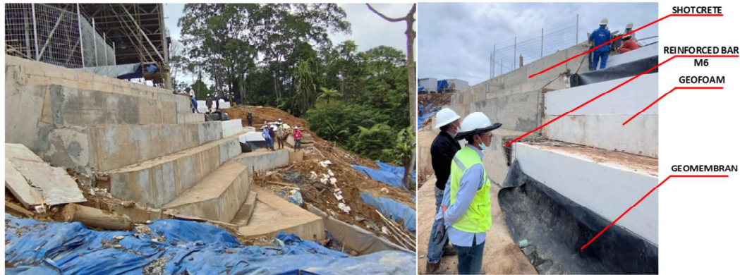
Figure 20. Geofabrication area –January 2023
