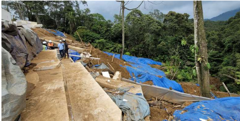
Figure 18. Geofoam installation area –December 2022
