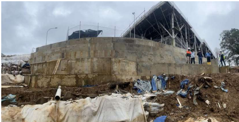
Figure 21. Geofabrication area –February 2023
