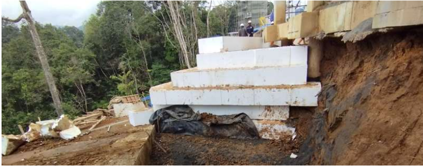
Figure 17. Geofoam installation progress – December 2022
