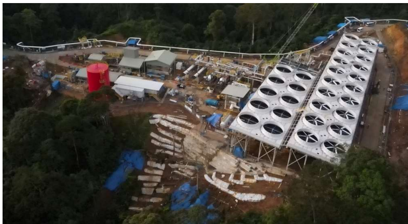
Figure 22. Access road and slope condition – May 2023
