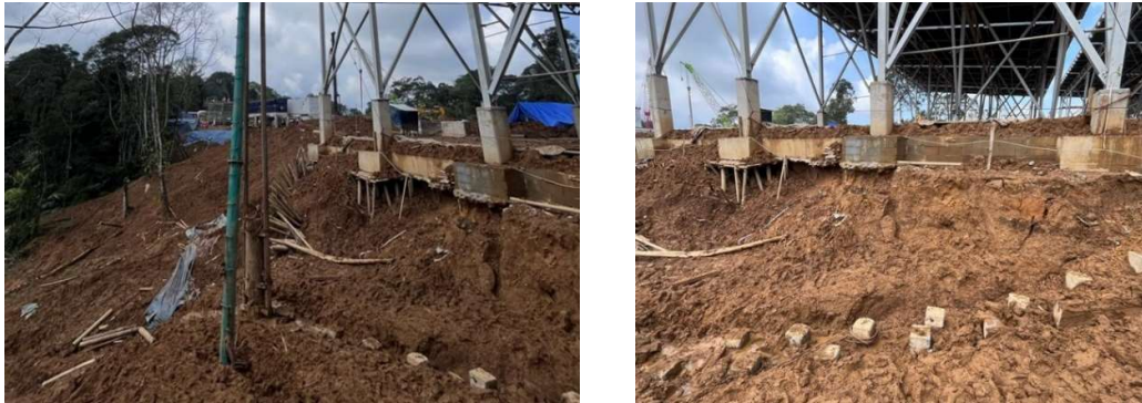
Figure 16. Slope condition on piling works area –October 2022
