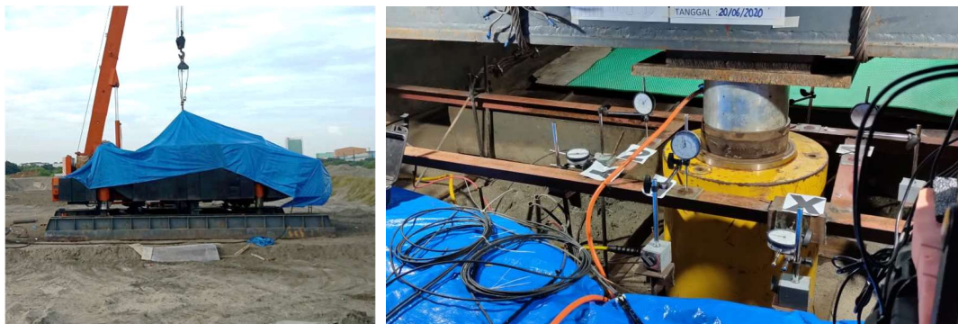
Figure 4. Load test on combine pile and cap/pad foundation (PT. GEC, 2020)
