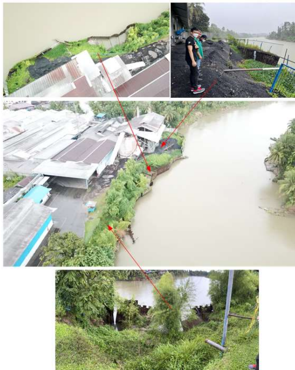
Figure 10. Sheet Piles Movement in 2022
