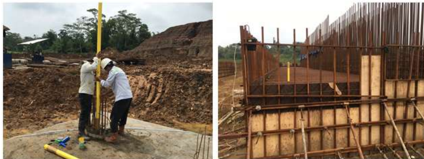
Figure 8. Inclinometer installation inside the spun pile
