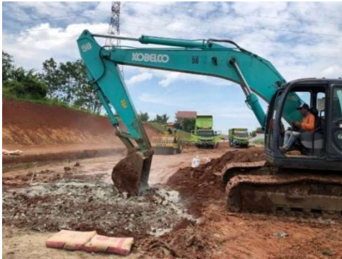
Figure 25. Soil cement was mixed using a backhoe
