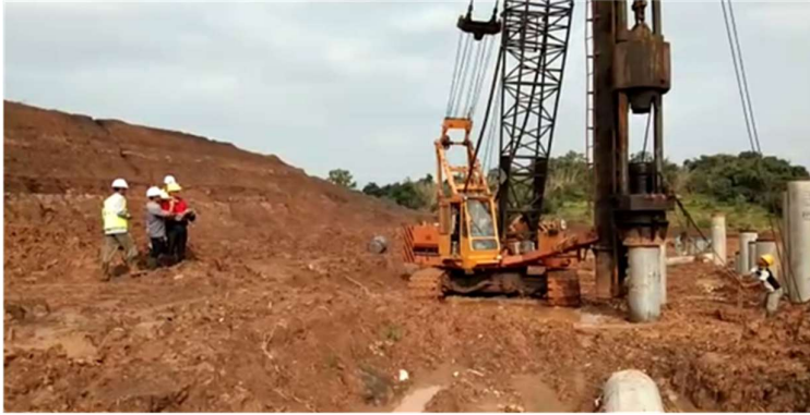
Figure 7. Documentation of pile driving process
