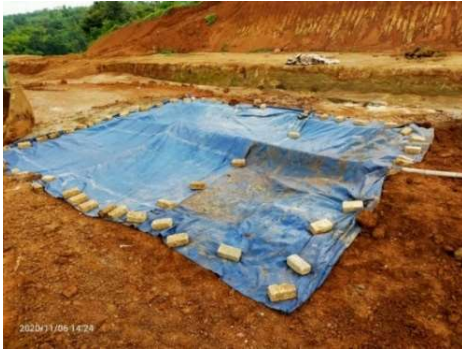
Figure 27. Curing process by covering the trial mockup area with a tarpaulin
