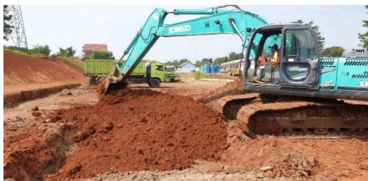
Figure 23. Selected lateritic soil is placed inside the trial mockup area
