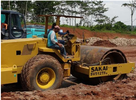
Figure 26. Soil cement compaction using vibro roller
