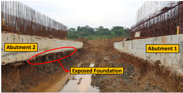
Figure 10. Documentation of exposed foundation after excavation was conducted between abutments
