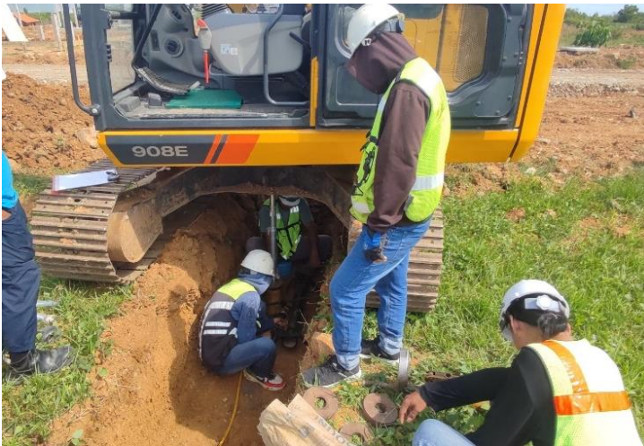
Figure 3. Excavator being used as reaction loading system for plate load test.
