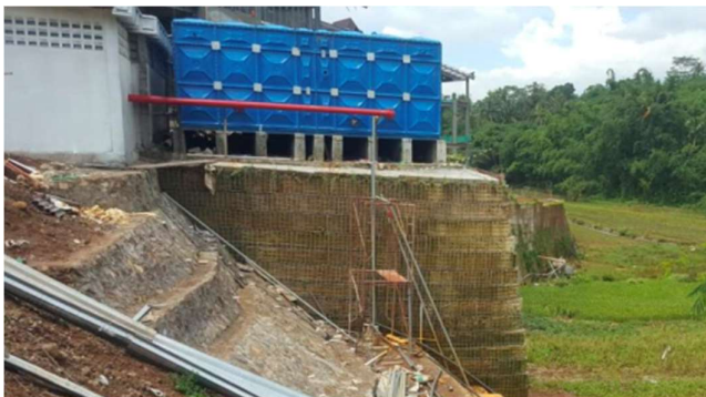
Figure 14. GWT structure in section 15 of KM 456 Semarang-Solo Rest Area
