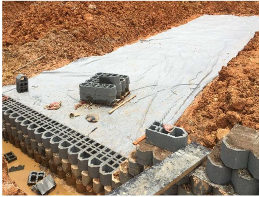
Figure 7. Installation of geocomposite reinforcement behind the reinforced soil wall
