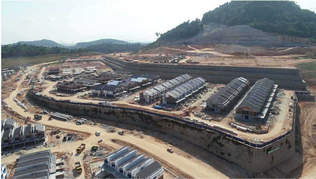
Figure 10. Overview of the reinforced soil wall
