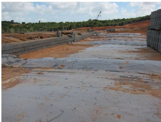
Figure 8. Drainage blanket and concrete drain incorporated in the reinforced soil wall
