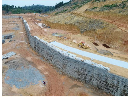
Figure 7. Installation of geocomposite reinforcement behind the reinforced soil wall
