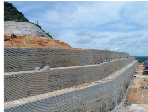
Figure 8. Drainage blanket and concrete drain incorporated in the reinforced soil wall
