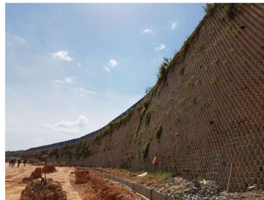
Figure 8. Drainage blanket and concrete drain incorporated in the reinforced soil wall
