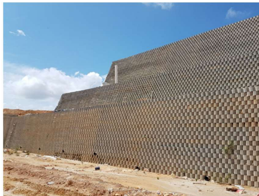
Figure 9. Completion of three-tier reinforced soil wall
