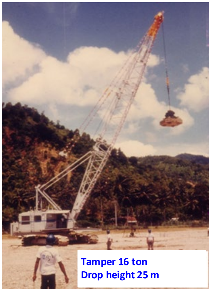
Figure 9. The documentation of dynamic compaction during tamping.
