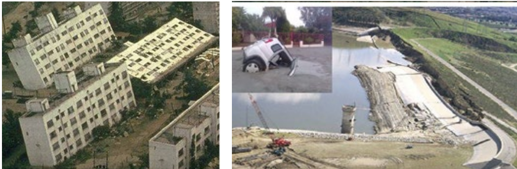
Figure 2. Destruction caused by liquefaction (Kramer, 1996; Geoengineer, 2015; López-Querol, 2008).
